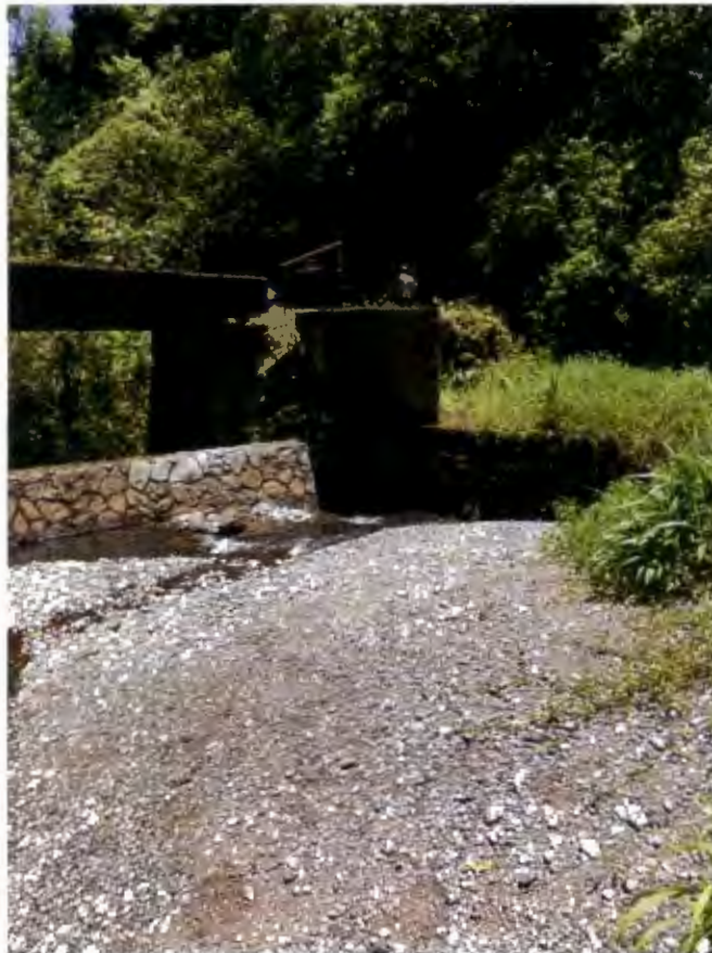
Figure 11. Dam, gate, and control structure at K-21.
