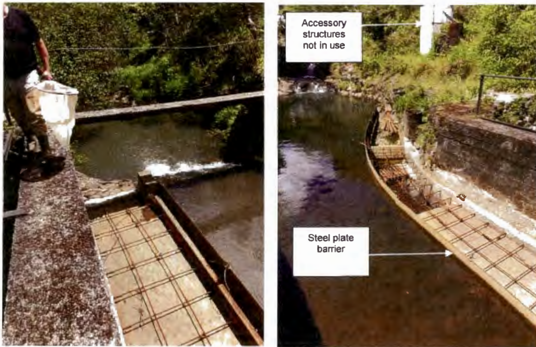
Figure 2. Grate to be sealed (left). Accessory pump house above grate (right).
